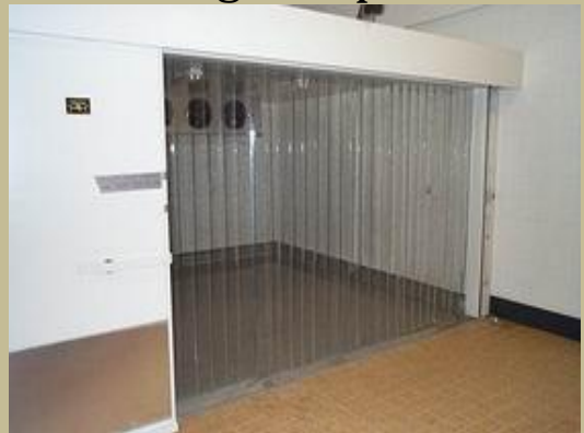
Pvc Curtains to retain Cool air in cold storage
