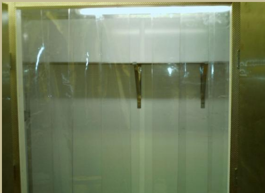
Pvc Curtains to retain Cool air in cold storage
