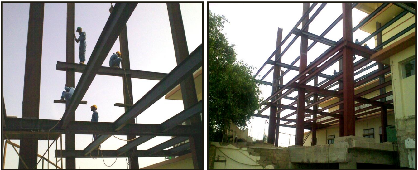
Figure 3: Steel Structure for School Extension
